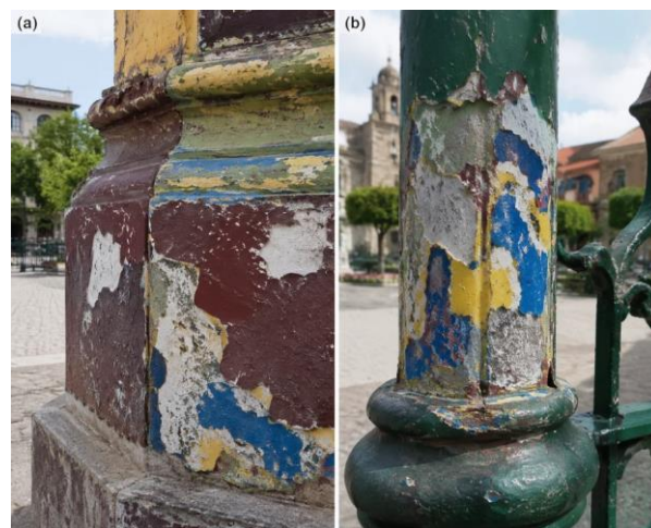
Figure 1. Multiple layers of paint with different colors can be observed on the same structure. Panel (a) corresponds to Site 01, and panel (b) corresponds to Site 02.
